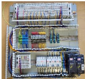
Figure 11: Electronics of the local crate with Beckhoff PLC for the motors.
